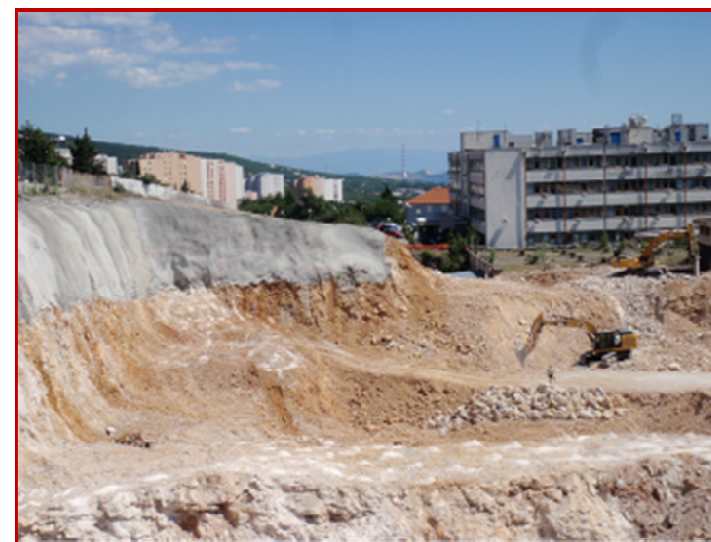
Construction Pit of the Future Hospital in Rijeka
